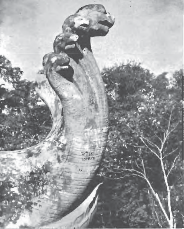
A naga balustrade.
