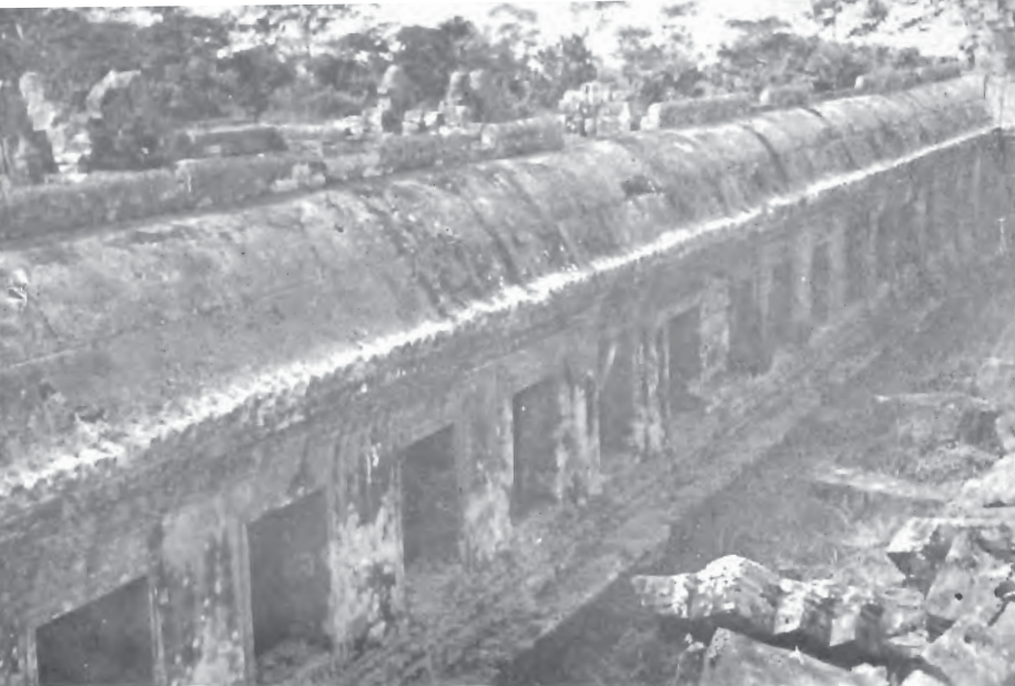
A south-western view of the galleries.
